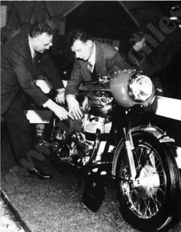
The short-lived headlight cowl that was an option for 1962 only and here seen fitted to a Matchless G12CSR Monarch of that year.
